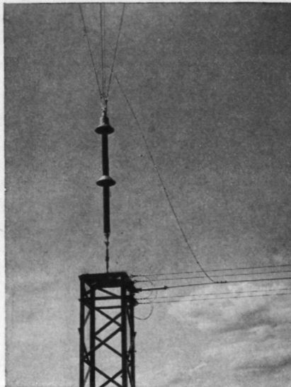
FIG. 1.41. Down-lead insulator and the end of the six-wire unbalanced unmatched feeder for the antenna of Fig. 1.5.
