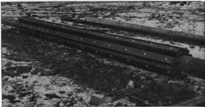
FIG. 3.111. A butt-spliced pole ready for erection. (Photograph courtesy of RCA Communications, Inc.)
